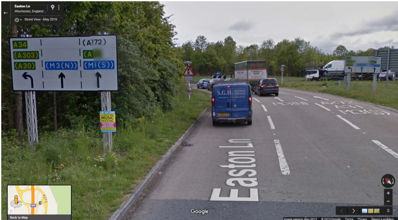
Above: Widened Easton Lane approach © Google 2015
